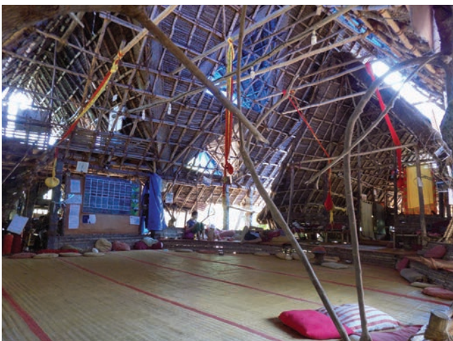
The main hut, in Auroville (Program Excursion), the structures all over campus are composed of organic matter and recycled products. There's an encompassing zero waste initiative.
