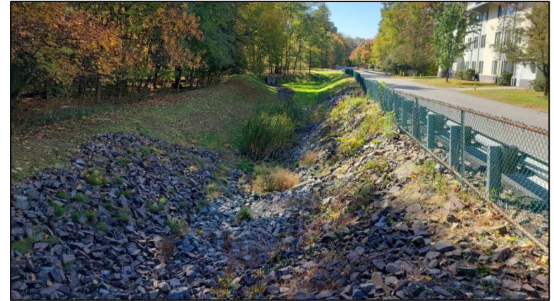
Detention Basin (store)
