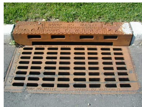
Catch basin near the parking garage
