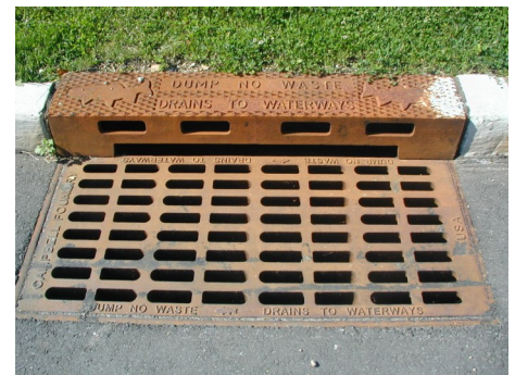
Catch basin near the parking garage
