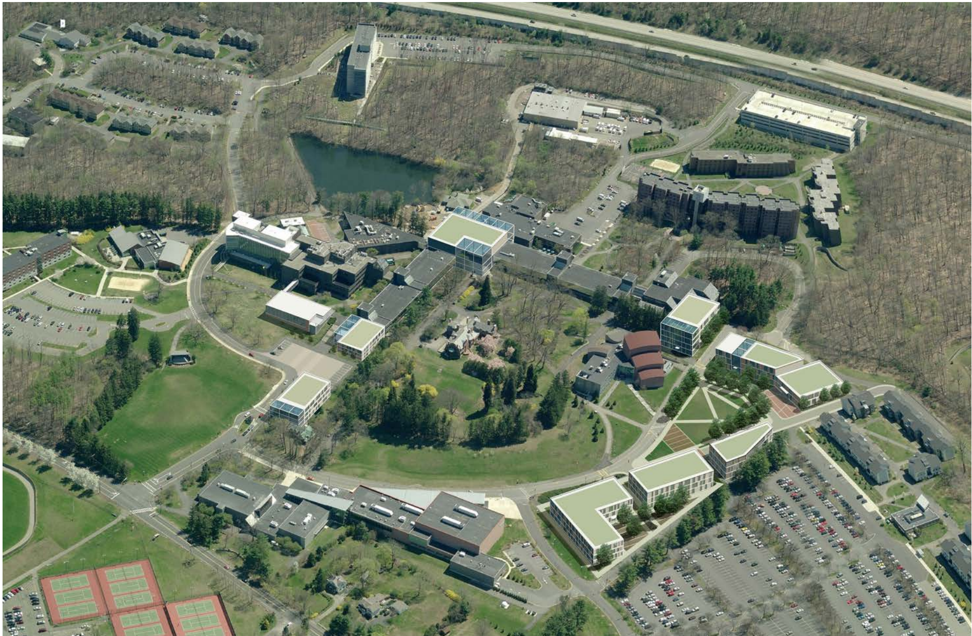
Figure 8B: Artist's rendering of the campus vision and potential evolution of the academic complex. Actual building design and footprints may vary.
