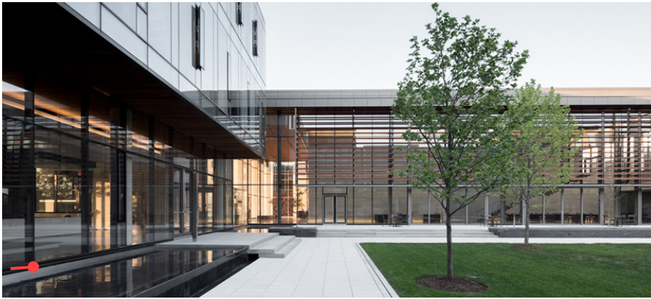
Building Envelop Transparency (CIGI Campus, Waterloo, Canada)
