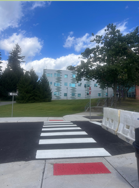
Crosswalk towards the Berrie Center.
